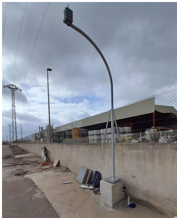
Figure 83: Detail of the metallic pole to keep the sensor box
